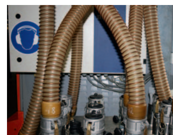
Hose station in the plastics industry
