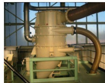
Transporting fritted glass filters
