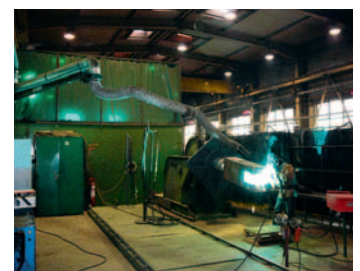
Welding smoke extraction
