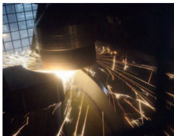
Extraction of welding smoke with increased flying sparks
