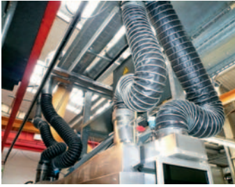
Extraction of aggressive chemical vapours during the manufacture of adhesive foils
